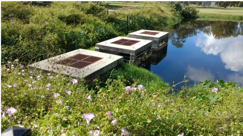
A **STORM** sewer system in which the flow receives little to no treatment prior to flowing into the river. Storm sewer lines are typically comprised of metal or concrete culverts and pipes, concrete or grass lined ditches, and catch basins (inlets).
